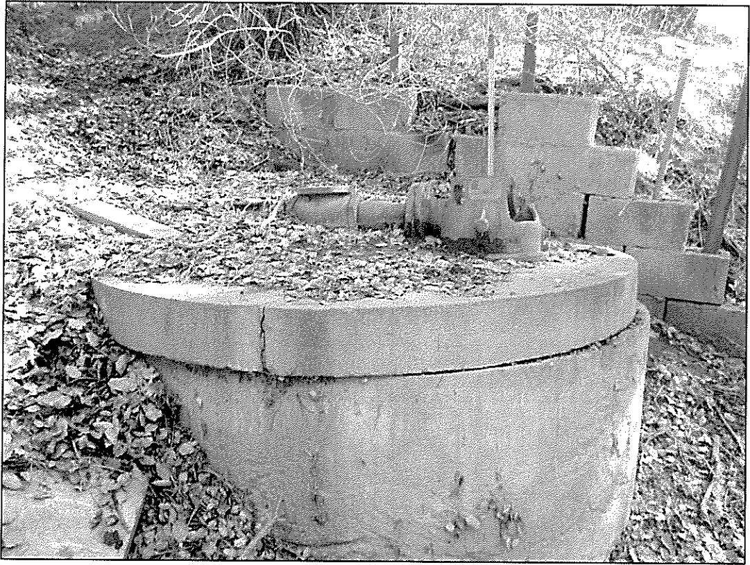
One of three on-site wells. This is one of two wells located in the trees by the flowing stream in southwest portion of the site adjacent Bear Valley Pkwy.
