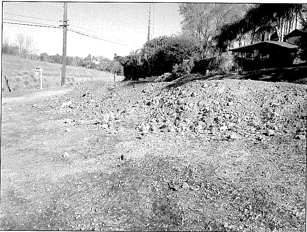
Suspected fill from unknown source extending over west berm of Choya Canyon Road at subject properties northern extent.
