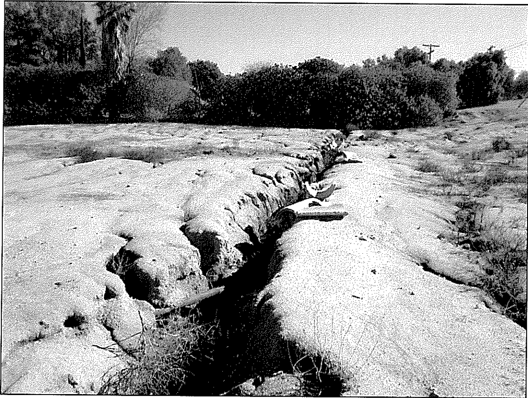
Typical deep surface erosion at isolated locations.
