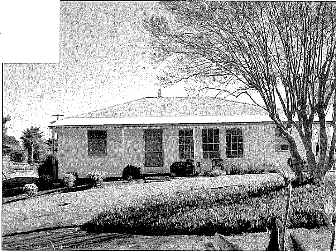
Three bedroom single story residence at 661 Bear Valley Parkway. Age estimated at 60 years. Escondido Building Department has no record of construction.
