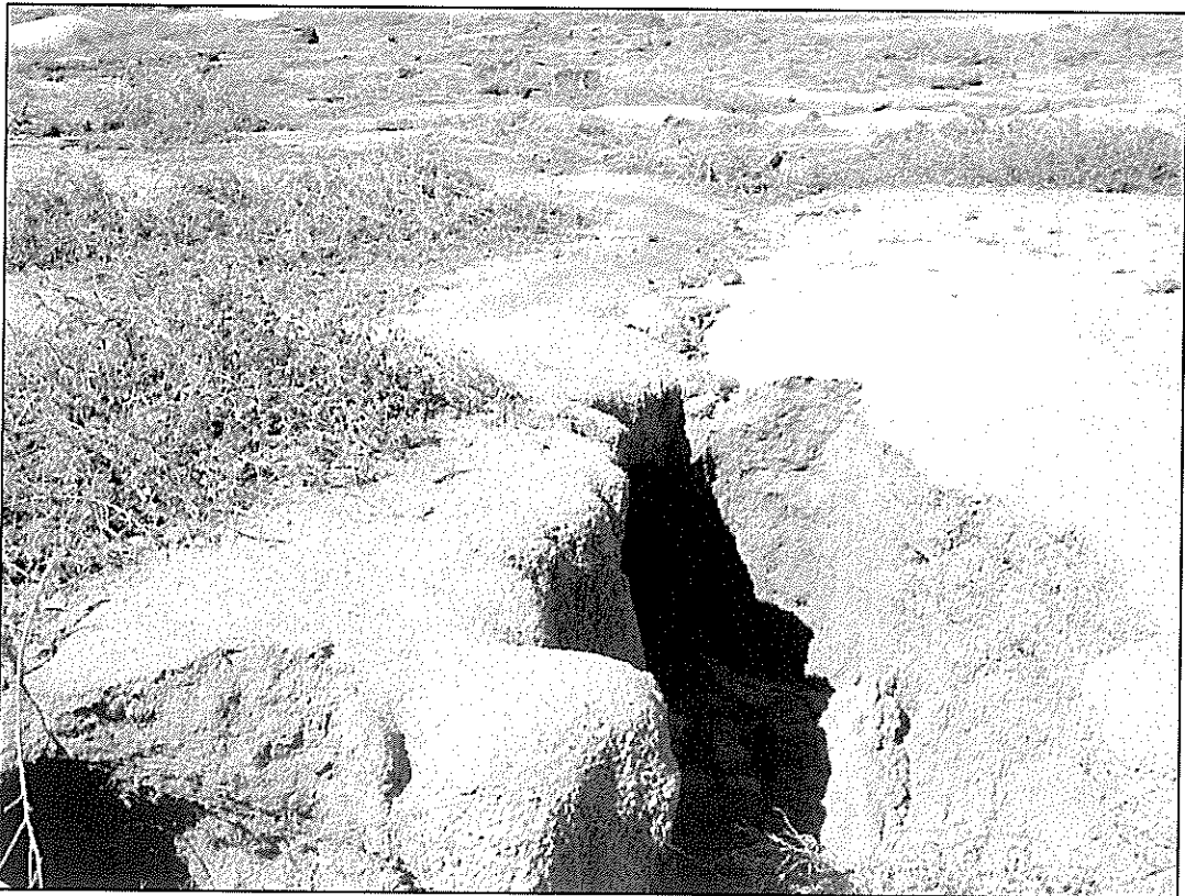
Note little erosion in background and severe abrupt erosion of same drainage.
